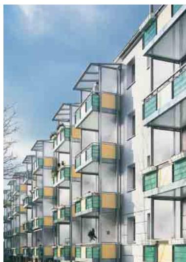
This free-standing balcony construction for later addition to buildings is held by supports in front of the façade and securely anchored to the building structure using fixing brackets. This is an ideal solution for total renovation:
