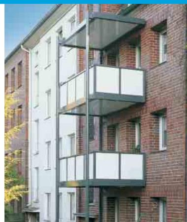
So-called balcony extensions are the most cost-effective type of balcony for improving suitable existing buildings. They are supported at the front by supports, whilst brackets are used on the wall side to attach them to the building.
